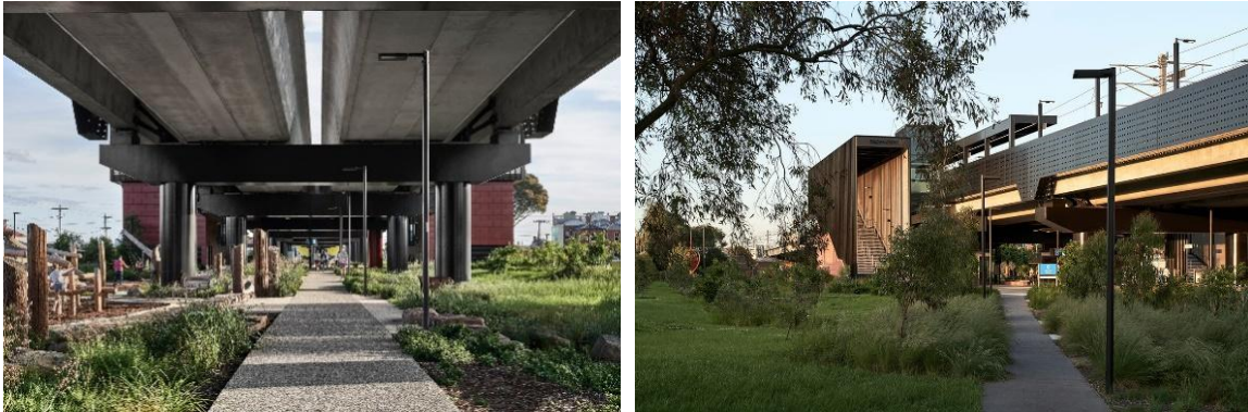
Bell to Moreland Level Crossing Removal Project / Brunswick and Coburg / Wurundjeri Woi-wurrung Country (2021) Architecture: Wood Marsh Landscape: Tract Photography: Peter Clarke
