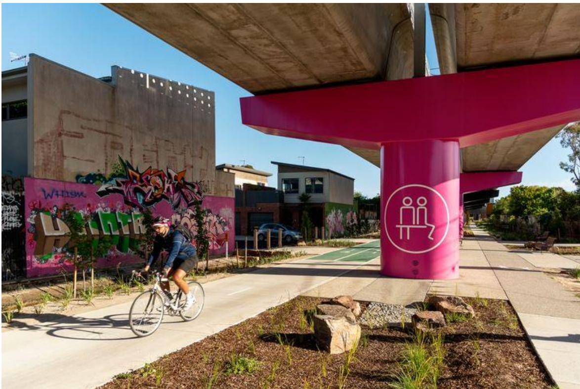
Bell to Moreland Level Crossing Removal Project / Brunswick and Coburg / Wurundjeri Woi-wurrung Country (2021) Architecture: Wood Marsh Landscape: Tract Photography: Robyn Oliver Photography Client: Level Crossing Removal Project (LXRP) OVGGA involvement: Chair, LXRP Urban Design Advisory Panel
