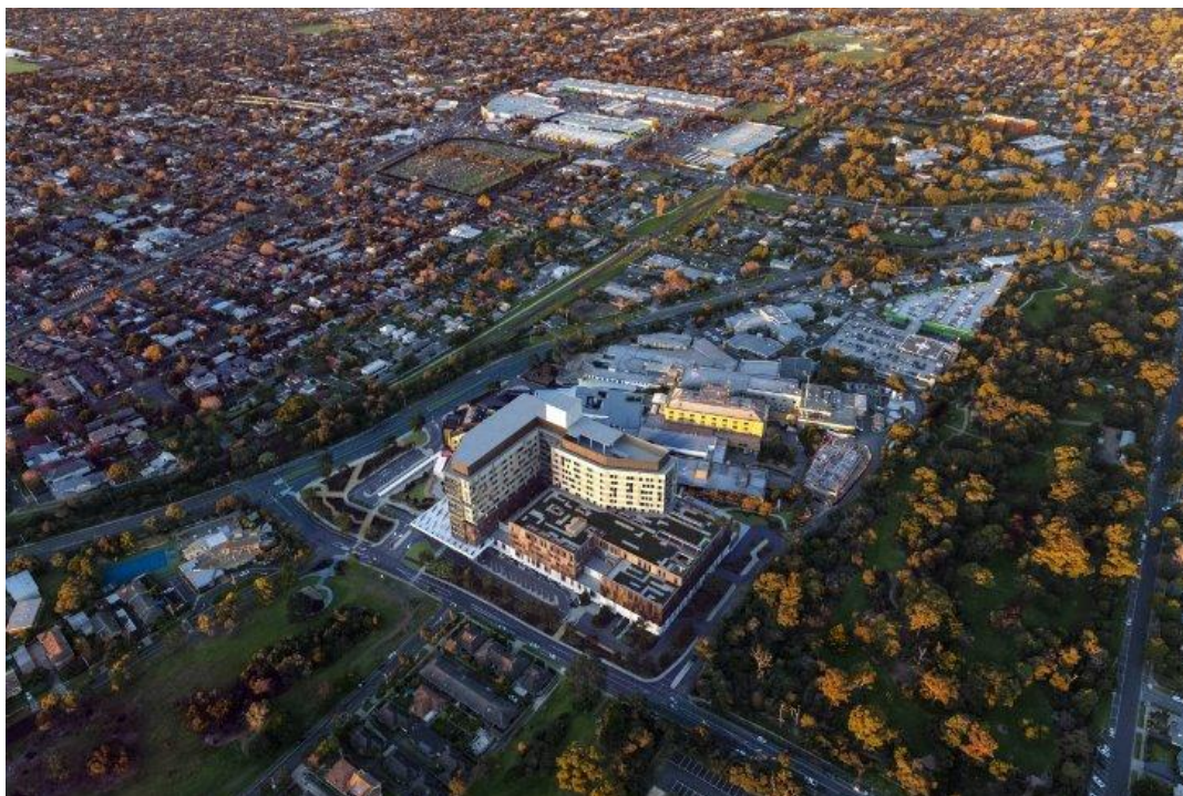
Architectural render of Frankston Hospital Redevelopment, Design team: Bates Smart + Architectus Conrad Gargett + Urbis
