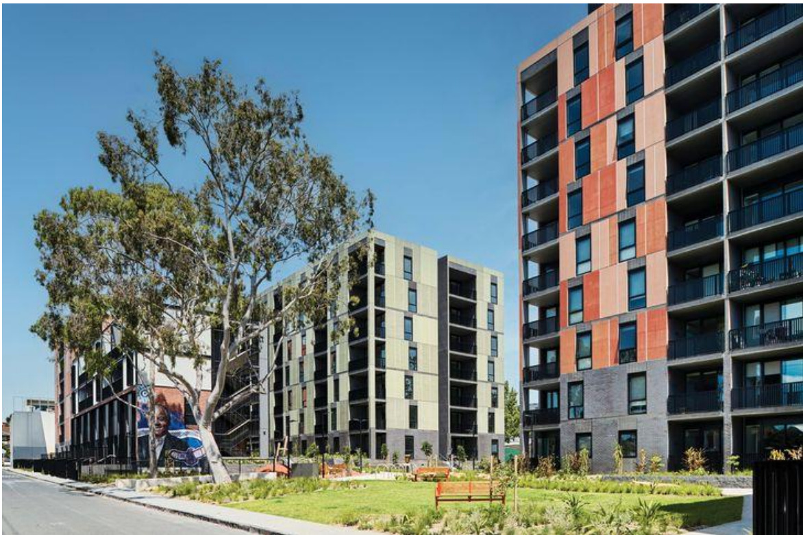
Bang Street, Prahran / Wurundjeri Woi-wurrung Country (2024) Architecture: Jackson Clements Burrows Landscape: Tract Photography: Tom Blachford Client: Homes Victoria OVGA role: Strategic advice, design review and tender evaluation during project procurement and delivery
